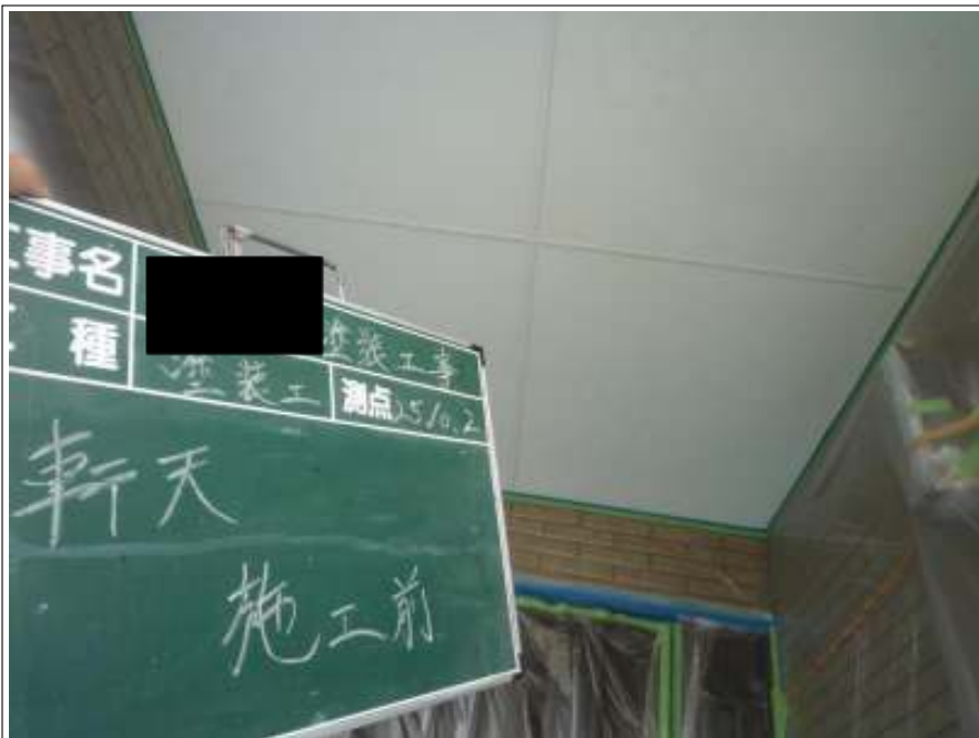
軒天塗装施工前
