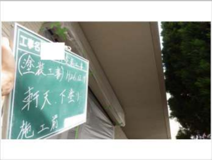
軒天塗装施工前
